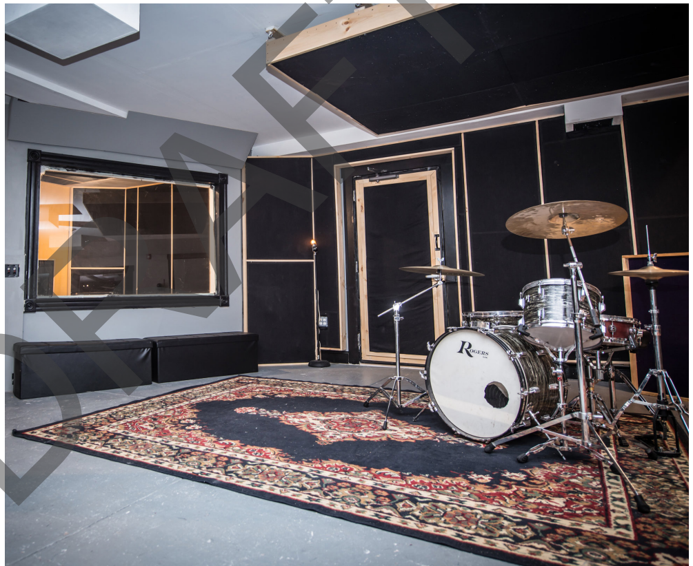
Right: Dead Moon Audio's recording studio located in the Armory basement.
