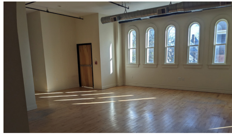
Right and Left: Vacant spaces in the Armory on the 2nd and 3rd floor
