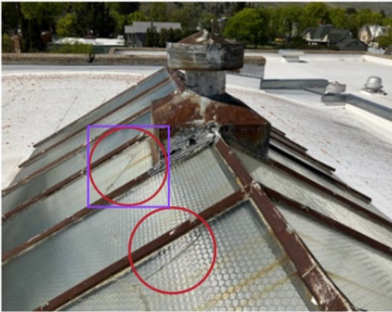
Additional Cracks
