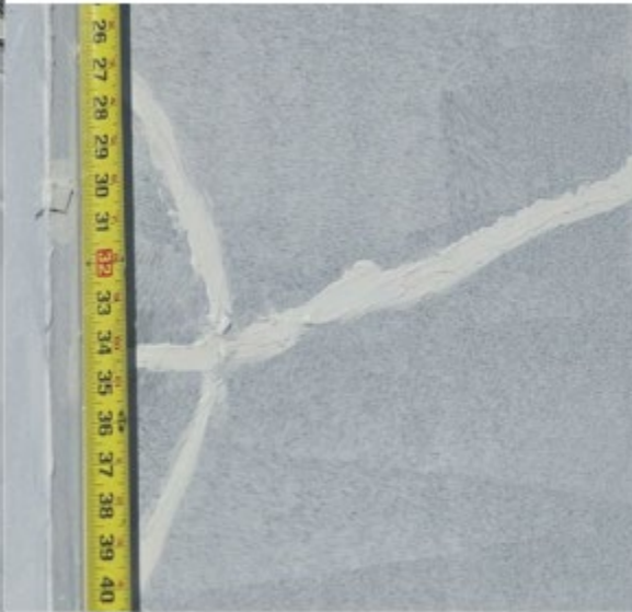
Measuring tape depicting the length of the panels and size of one portion of a crack with elastomeric
