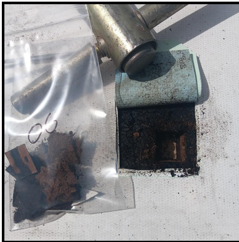
ASBESTOS Sample 06 old roofing ASBESTOS
