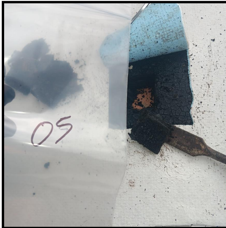
ASBESTOS Sample 05 old roofing ASBESTOS
