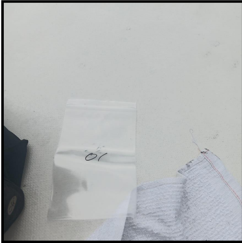
Sample 01-03 roofing New Roof
