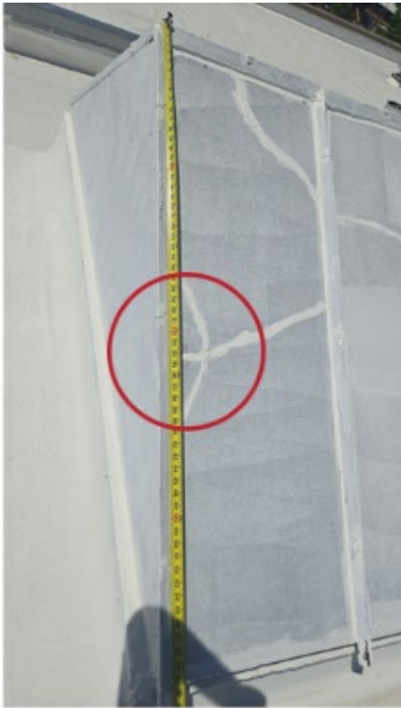
Measuring tape depicting the length of the panels and size of one portion of a crack with elastomeric
