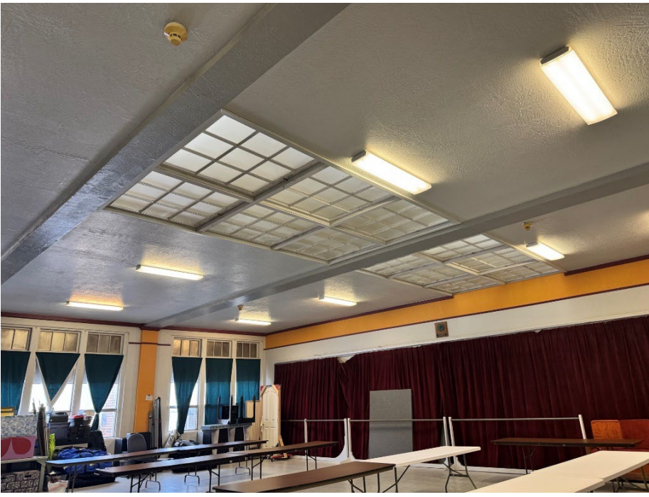
3rd Floor Community Room with Interior Skylights
