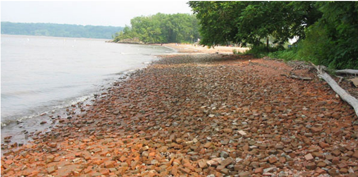
The brick filled beach at Kingston Point (existing)
