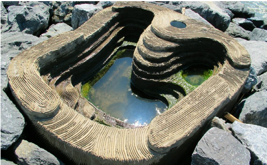
Eco-concrete units (proposed)
