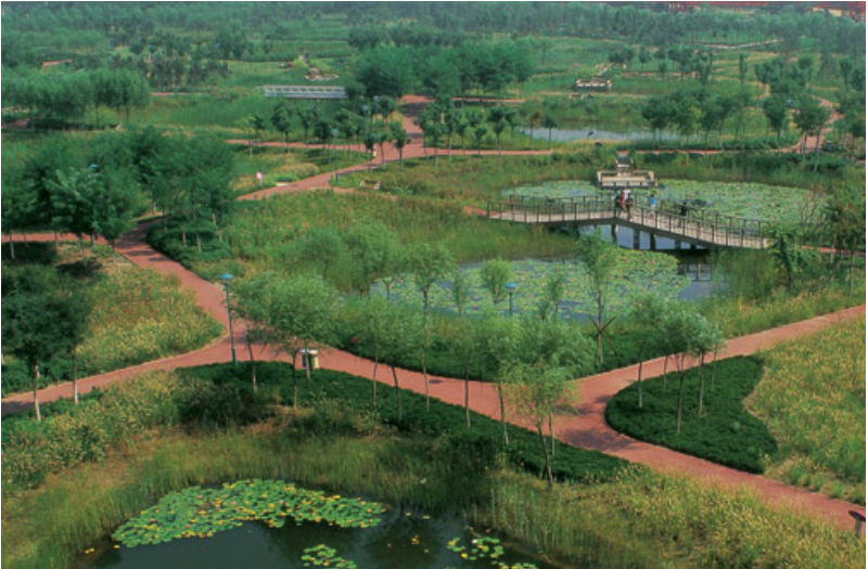
Stormwater retention park
