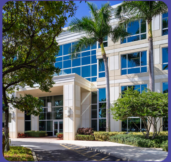
Main entry of existing facility.
