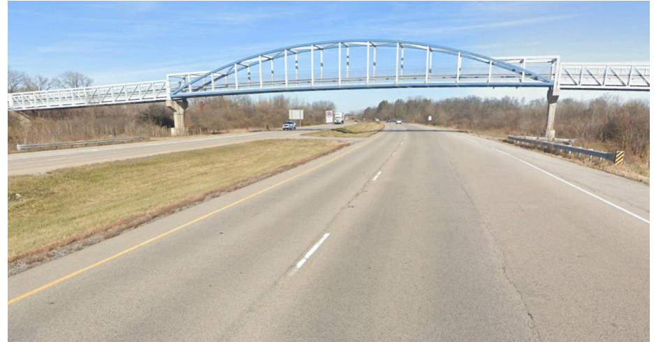
Pedestrian and bicycle bridge along the Virgil Gilman Trail over Highway 56. Photo Credit: Design Workshop
