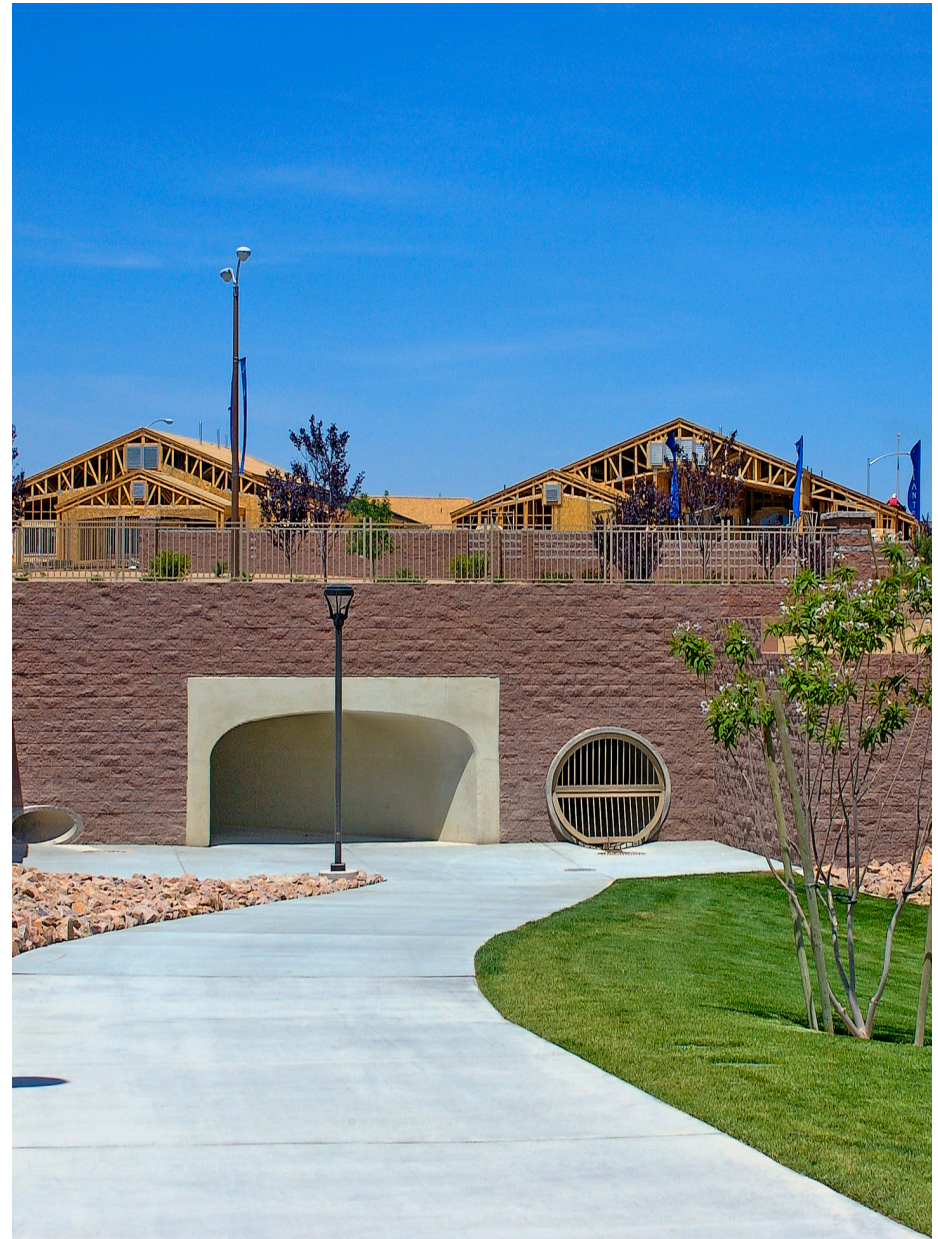
An example of a pedestrian and bike bridge under a busy road. Photo Credit: Design Workshop
