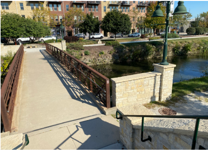
Pedestrian bridge across the Canal
