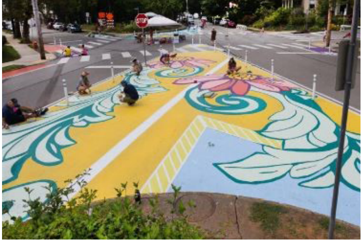
Painted pavement treatment
