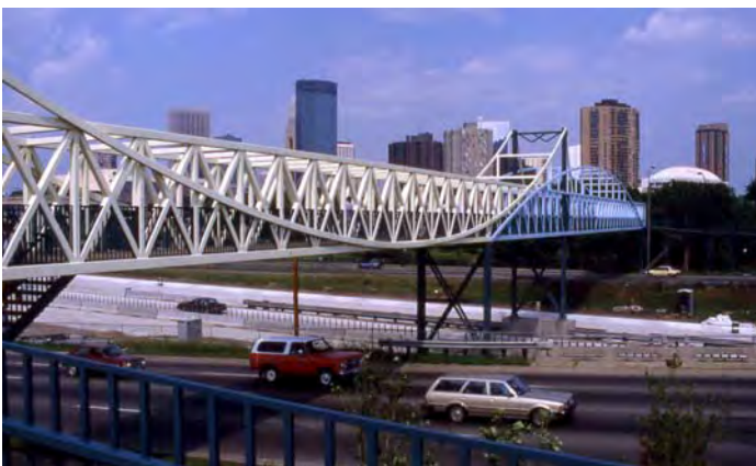
Steel Truss - Minneapolis
