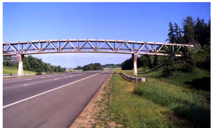
Wood Truss - St. Cloud
