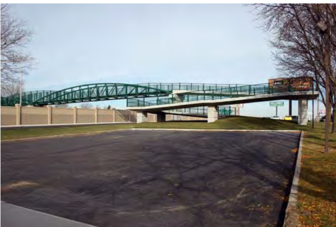
Arch Truss - Rochester
