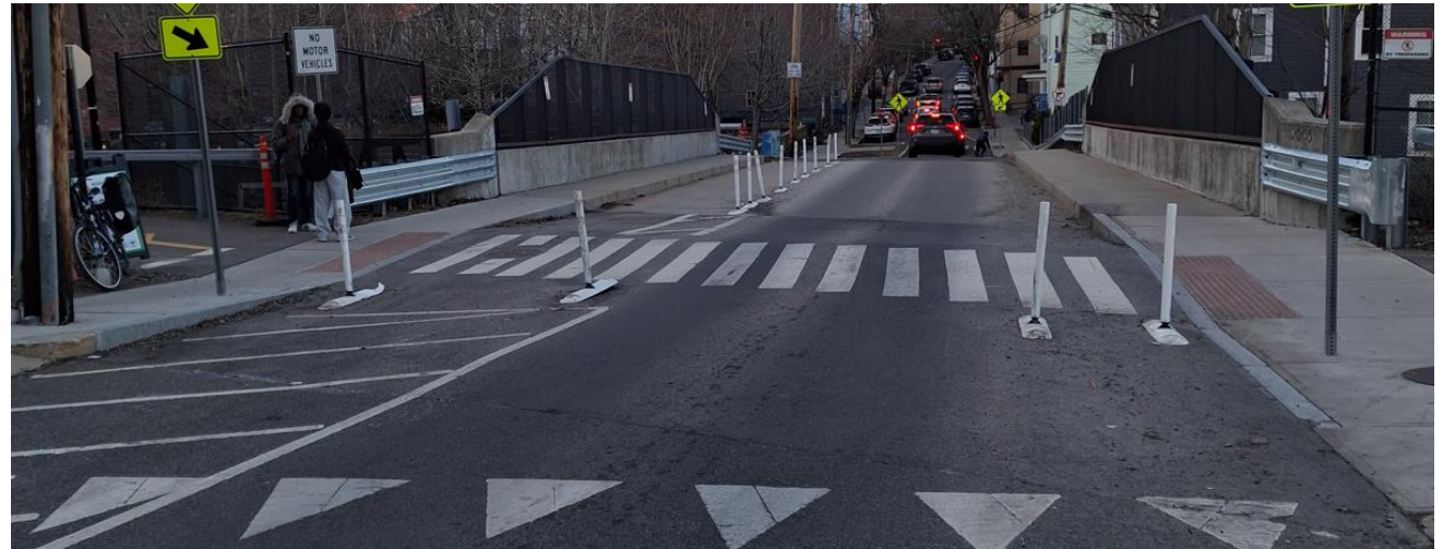
Existing temporary installations at Sycamore and Walnut
