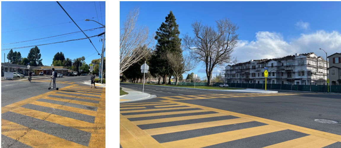
FIGURE 15 MARKED CROSSWALKS IN MOUNTAIN VIEW
