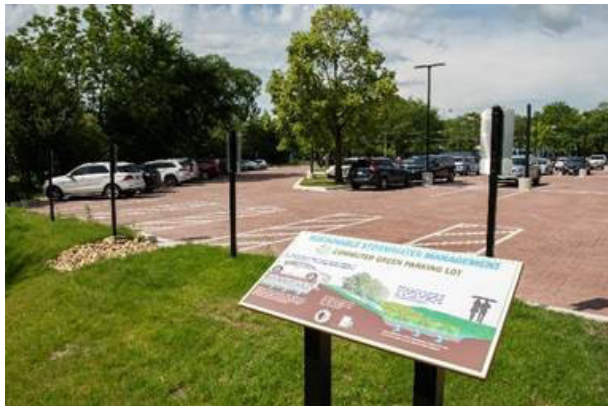
Parking lot with permeable pavers
