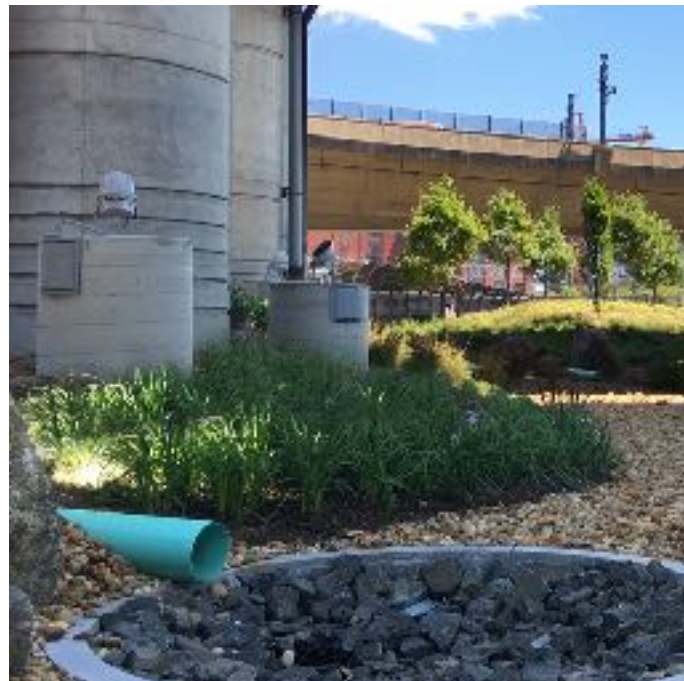
Underground at Ink Block drainage swale
