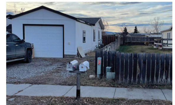
Blocked Access Easement
