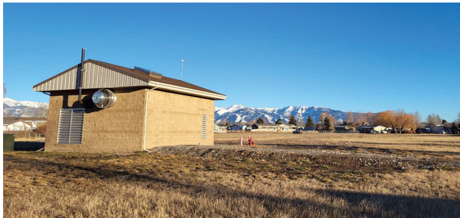
Existing Well Pump House
