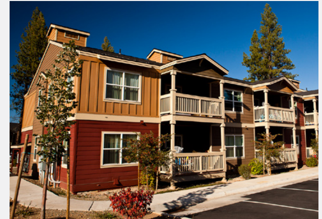
Henness Flats Apartments (approximately 14 dwelling units per acre.)
