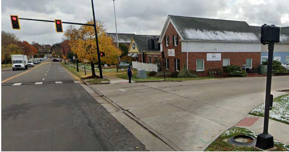
Figure 7: Segment – Hudson Plaza Shopping Center (West Entrance) Pavement Condition
