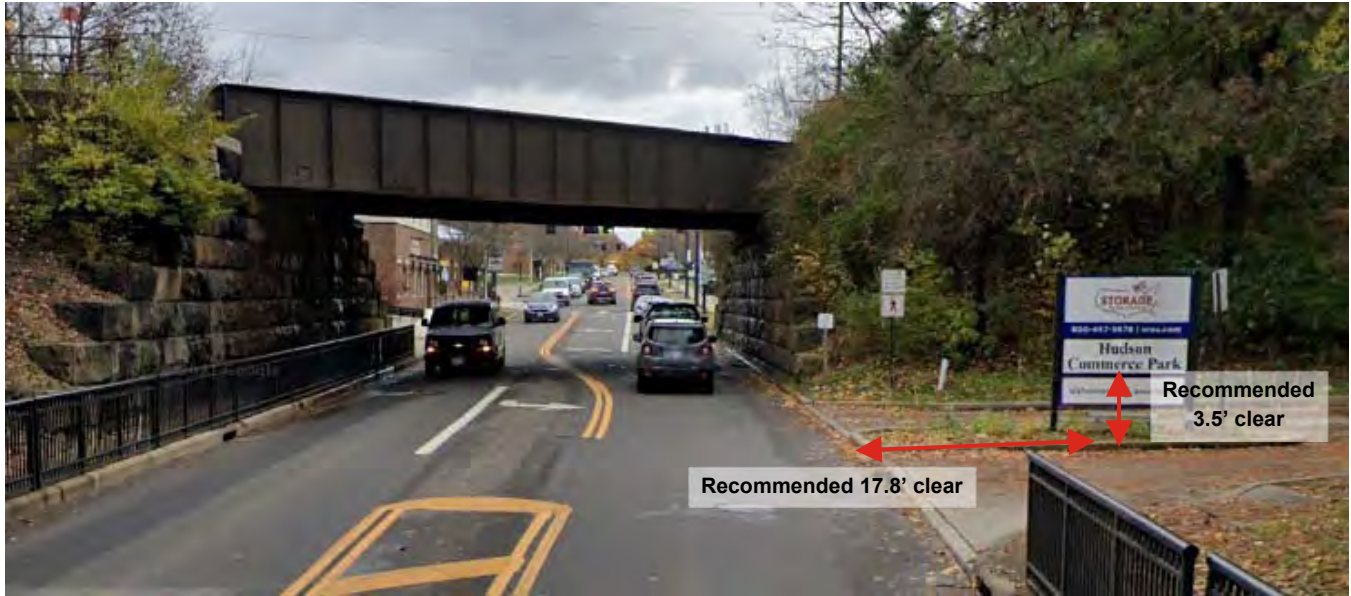
Figure 4: Sign blocking sight distance
