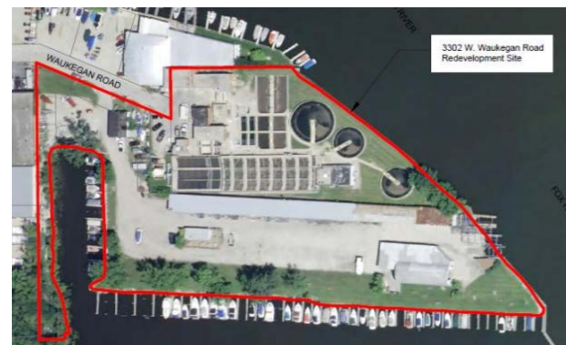
Figure 3.2. City of McHenry's former wastewater treatment plant.
