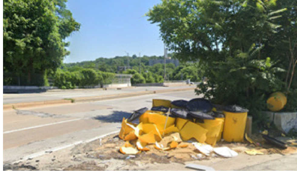
Damaged crash barrels at Northern Parkway and I-83
