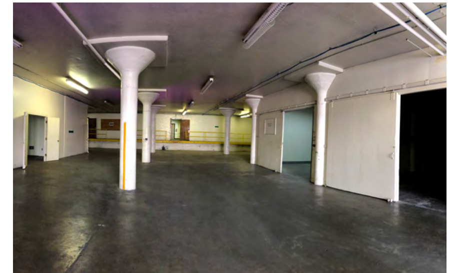
FIGURE 12. Mushroom column at lower level
