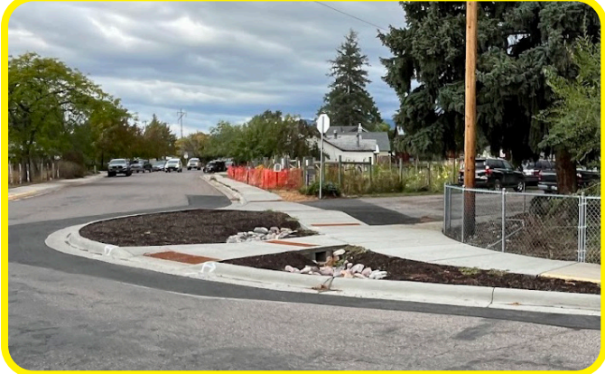
Traffic calming and management at intersections: permanent and quick-build traffic circles are one example. Others include bulb-outs. No center line markings, sidewalks on both street sides, tight curb radii, and unmarked crosswalks are also characteristic typical treatments of Neighborhood Residential streets.
