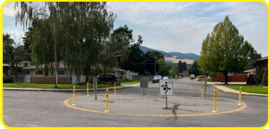
Traffic calming and management at intersections: permanent and quick-build traffic circles are one example. Others include bulb-outs. No center line markings, sidewalks on both street sides, tight curb radii, and unmarked crosswalks are also characteristic typical treatments of Neighborhood Residential streets.
