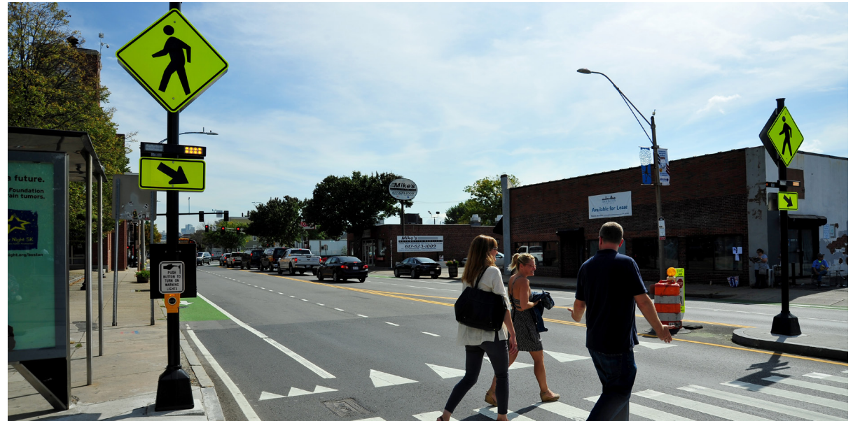
FIGURE 5-23 Rectangular Rapid Flashing Beacon (RRFB)
