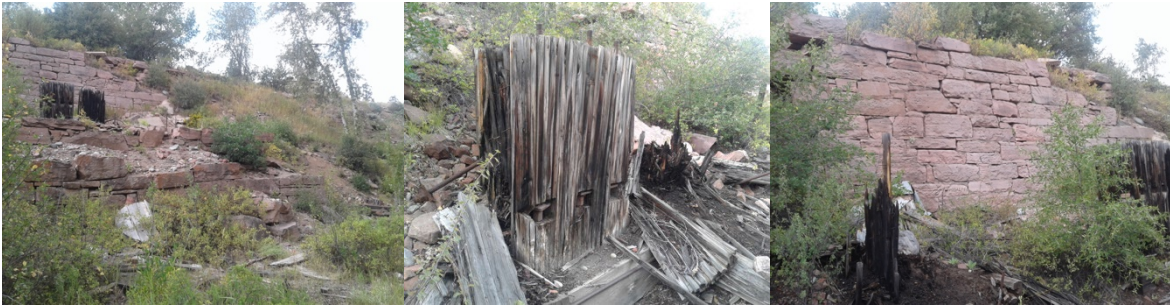
28 Sandstone foundations and walls, and wooden stamp piers that are part of the ruins of the historic Holden Lixiviation Works
