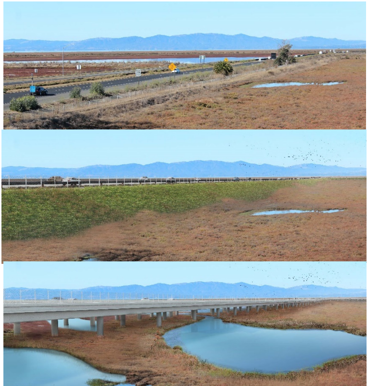
Sea level rise strategies for SR 37, which runs along the northern shore of San Pablo Bay to the north of San Francisco (top: current condition; middle: proposed embankment; bottom: proposed causeway). Images courtesy of Metropolitan Transportation Commission.
