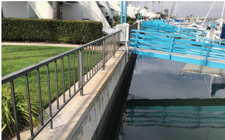
4. Coronado Cays bulkhead with a small freeboard between the high tide line and the ground surface
