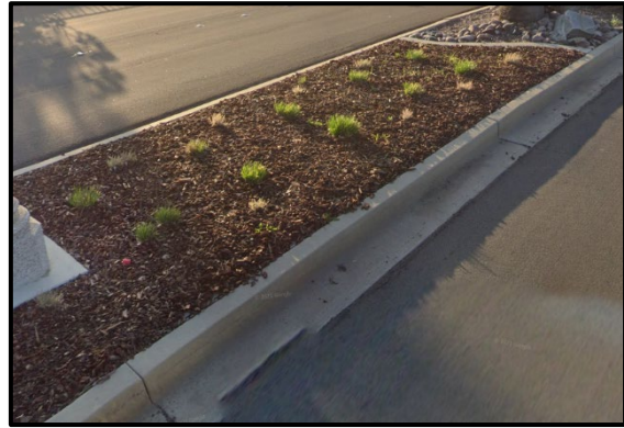
Figure AP-57: Permeable medians, such as this one along Coronado Cays Boulevard, can help reduce flooding on streets
