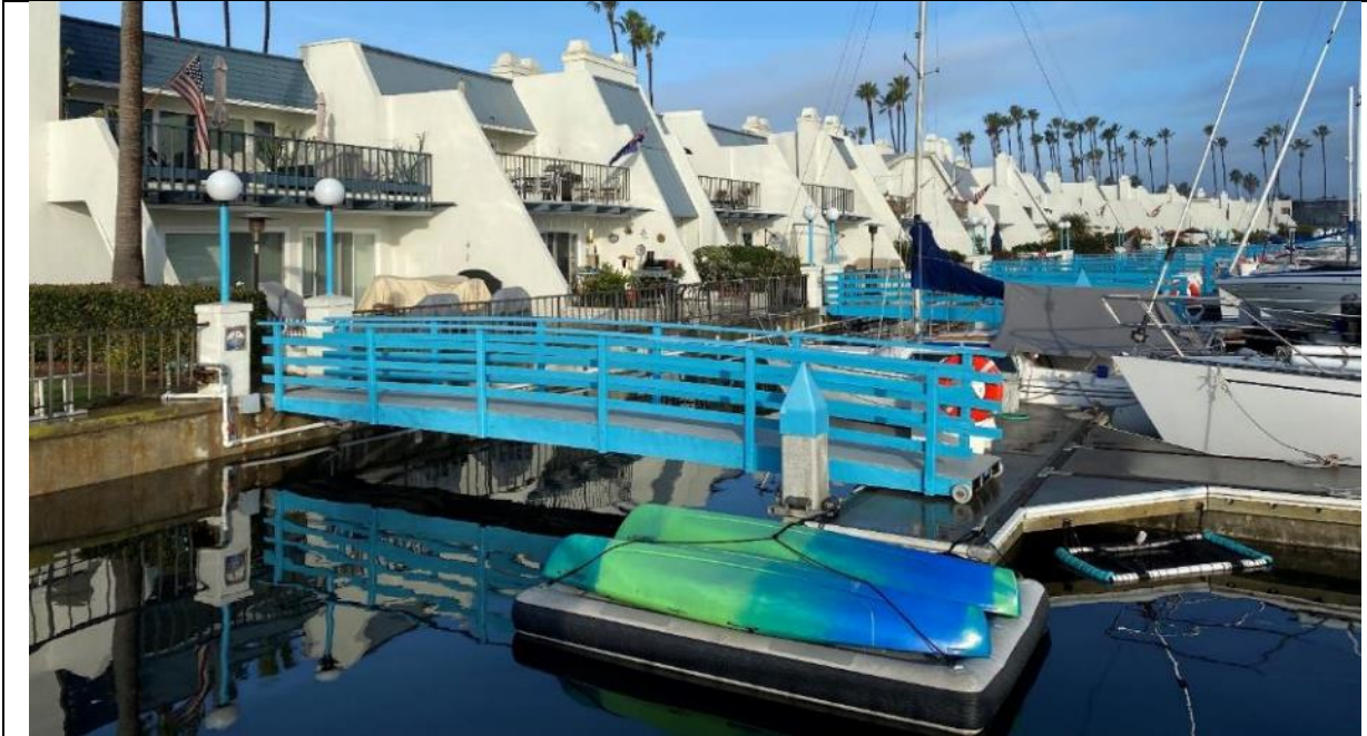
1. Gangways and piles near their functional limit during December 2020 king tide
