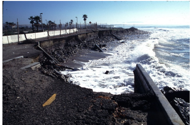
Surfers' Point Park in Ventura, CA has experienced repeated damage from coastal erosion. Image courtesy of Surferspoint.org.
