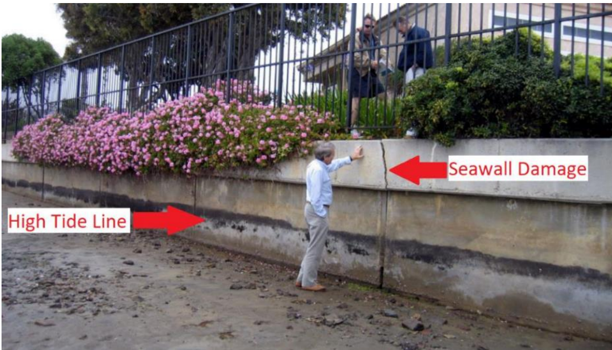
6. Bay-side photo of Coronado Cays showing bulkhead seawall damage
