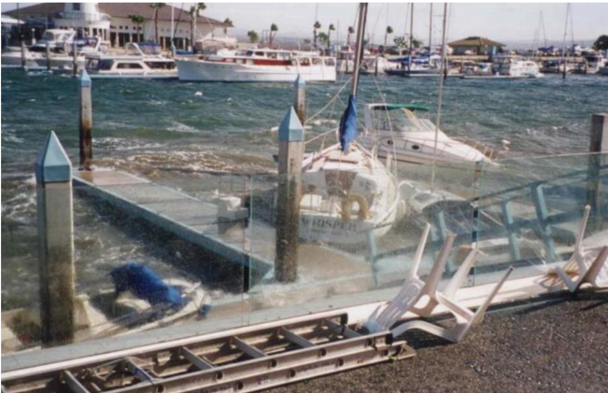
2. Wave damage at Coronado Cays Marina during Santa Ana wind event
