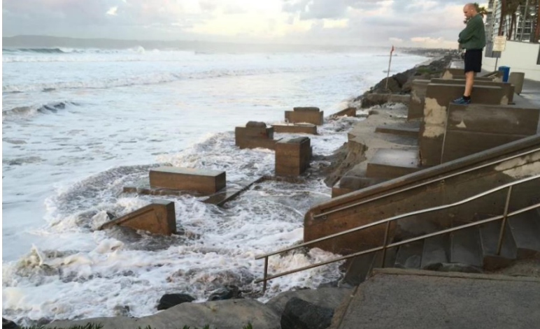
2. Wave runup at the Coronado Shores revetment and beach access ways (Voice of San Diego 2016)
