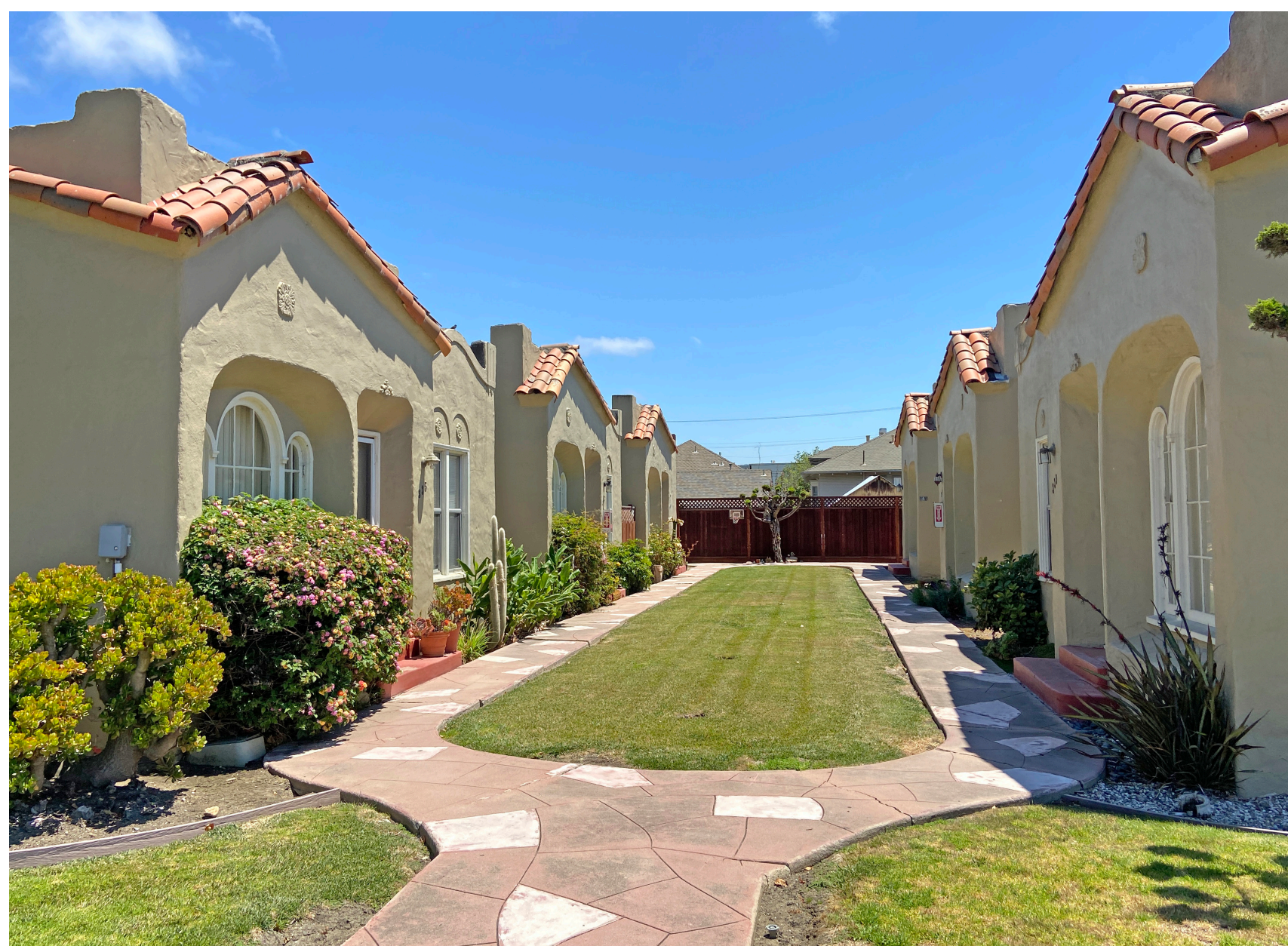
Bungalow court – Riker Street Cancha Bungalows – Riker Street
